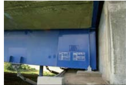
Photo 1. After Partial Repainting
