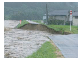
Washout of a dam due to erosion by running water
