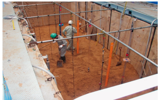
写真-2 試験地盤作成状況 Photo 2 Construction of the experimental ground
