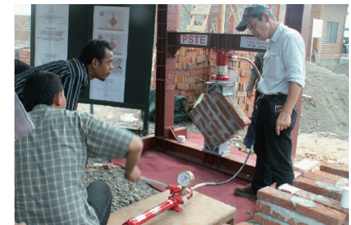
Fig. 6 Test by a foreman (mandor)
