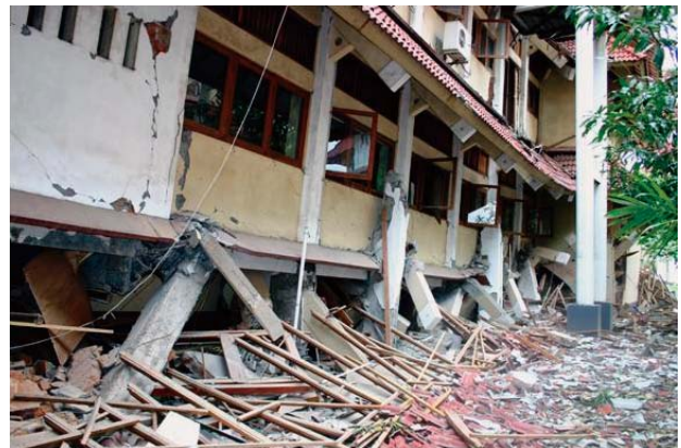
Photo 2 Damage to reinforced concrete building
