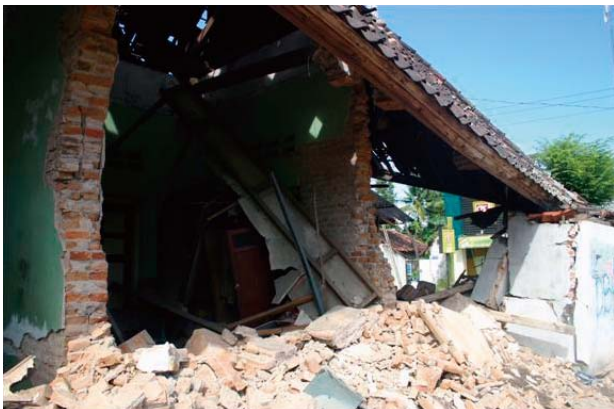
Photo 1 Damage to unreinforced concrete building
