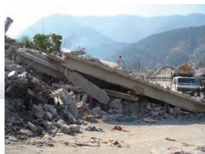
Photo Collapse of 1- or 2-storey RC building in Balakot
