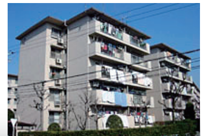
Photo 2 Adding rooms on the south of a building
