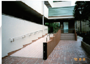
Photo 1 Construction of a slope with an appropriate inclination along entrance stairs and better-grade finish of the approach
