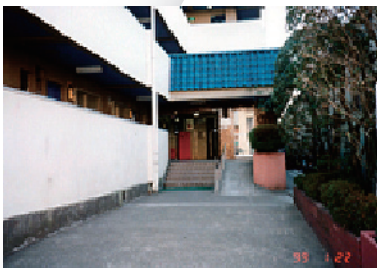
Photo 1 Construction of a slope with an appropriate inclination along entrance stairs and better-grade finish of the approach
