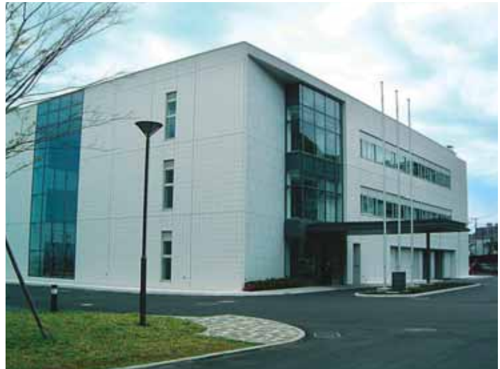
Full view of the new offices (Full view from the entrance side)
