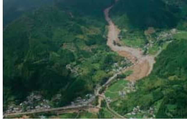
Photo 1 Debris flow which occurred in the Houkawachi-Atsumari District of Minamata City in Kumamoto Prefecture (Full View)
