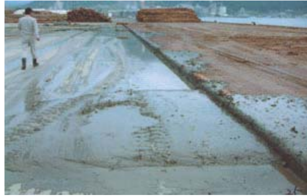
Photo 2 Deposit of silt erupted out behind a pier
