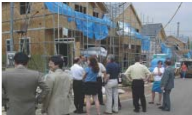
Photo 4 Technical tour to construction site
