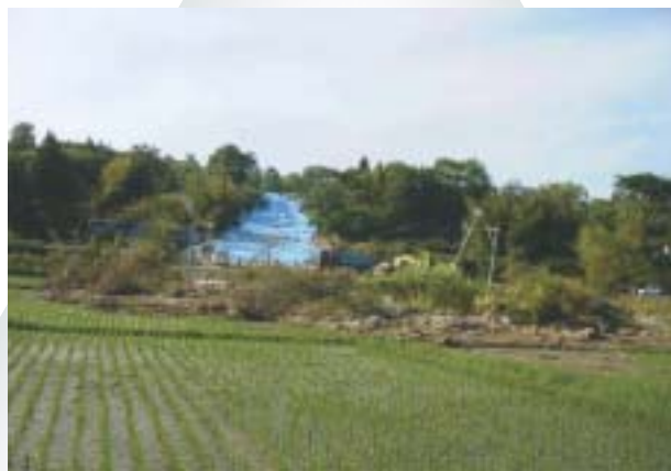
Photo 1 Large-scale flow slide of a banked slope
