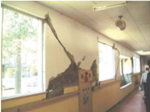
Photo 3 Damage to the corridor wall of a primary school building
