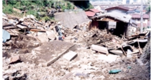
Photo 3 View of the destroyed houses (July 12, 2002)
