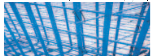
Damage prevention work against salt attack (steel bars coated with epoxy resin)
