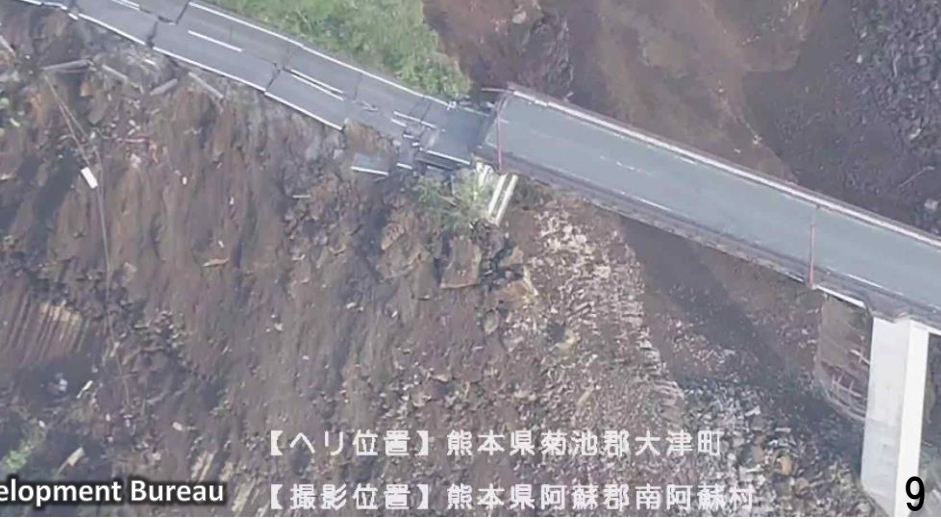
Damaged bridge (Choyo Bridge) 九州地整はるかぜ号
