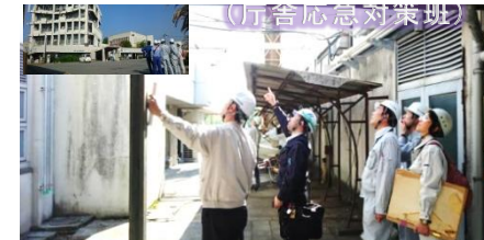
▼ Emergency safety assessment of a damaged building
