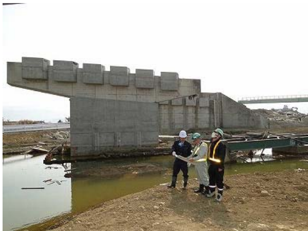
(a) Numata Overpass
