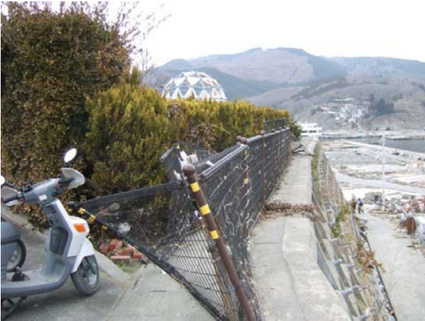
Photo 3.3.1.21 Steel bars and hedge on the east side of the hill
