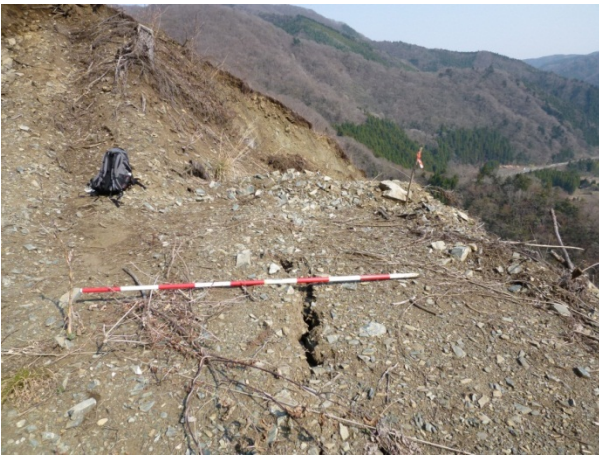
Photo 3.3.1.32 A crack seen on a strip road at the left side of the slope
