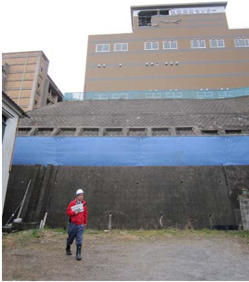
Photo 3.3.1.6 Retaining wall, cribwork, block pitching work
