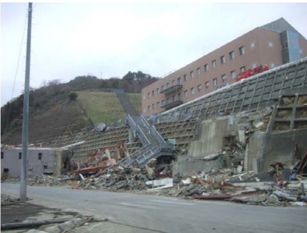
Photo 3.3.1.22 A steel stairway for evacuation from tsunamis
