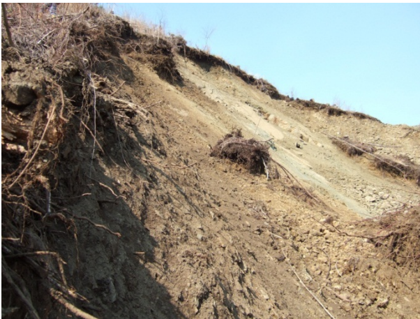
Photo 3.3.1.24 An upper portion of the collapse (an exposed rock is seen at the center)
