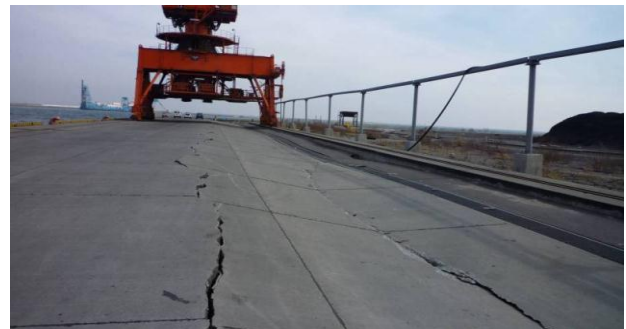
(a) Pier no. 3
