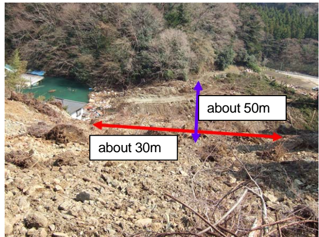
Photo 3.3.1.33 A blocked river channel seen from the center of the collapsed slope
