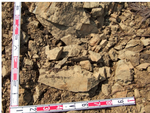
Photo 3.3.1.28 Collapsed sediment at the terrace
