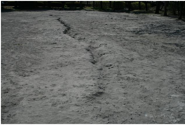
(a) Crack generated on the ground of a square
