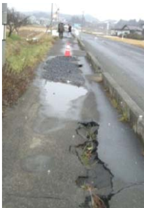
Photo 3.3.2.6 Conventional construction (without any anti-liquefaction measure)
