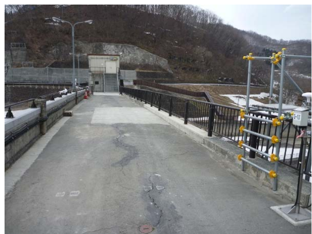
Photo 3.3.4.4 Crest of the Ishibuchi dam (3.11 earthquake)
