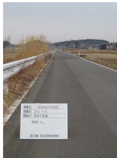
Photo 3.3.2.4 Construction subjected to the anti-liquefaction measure (no damage)
