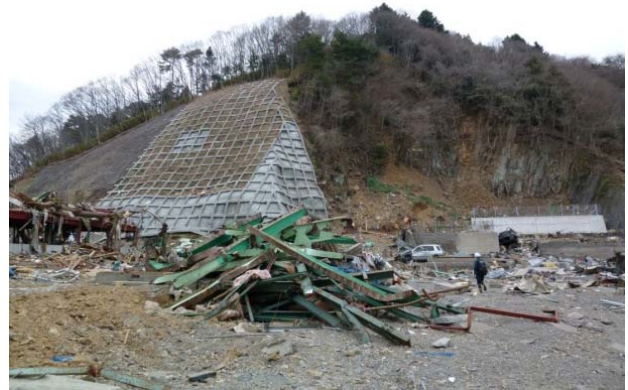
Photo 3.3.1.8 Earth falls on the right side of the cribwork (Onagawa)
