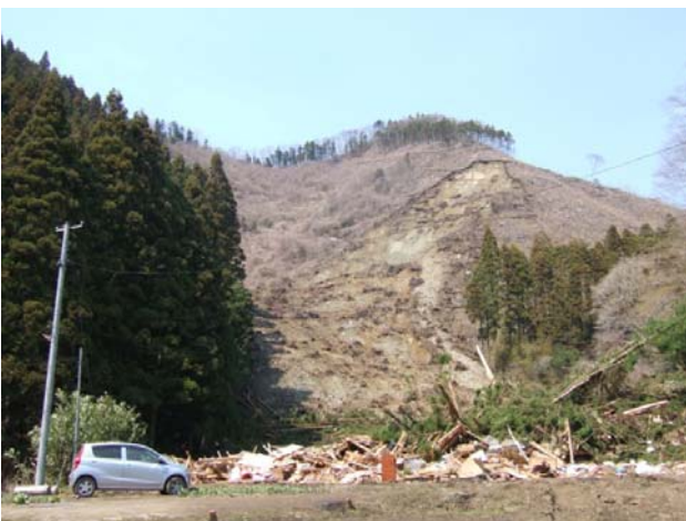
Photo 3.3.1.23 A whole picture of the slope failure
