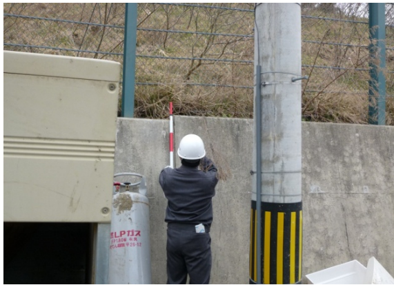
Photo 3.3.1.10 A dip slip of the retaining wall
