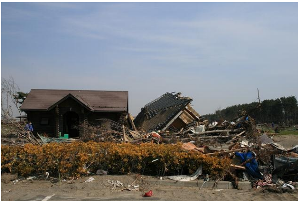
(a) Damage of Facility
