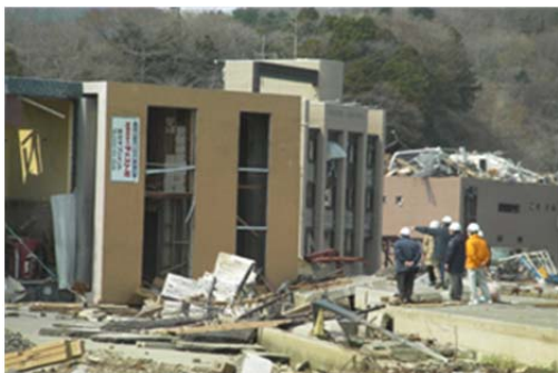
Photo 3.3.9.15 Field Survey by Building Construction Standards Association (Onagawa Town)
