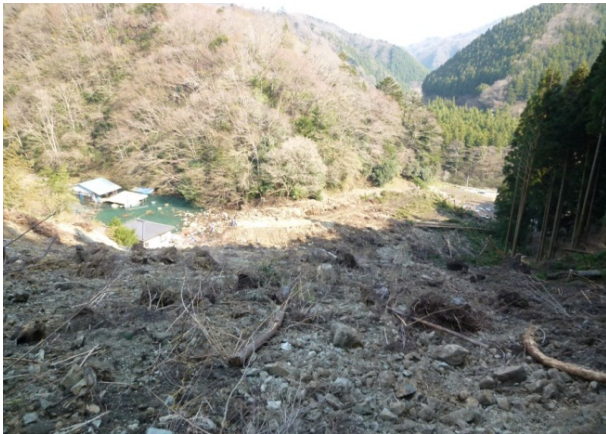
Photo 3.3.1.27 Sediment reaching a house (seen from the terrace at the center of the slope failure)
