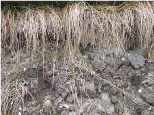
Photo 3.3.1.17 A zoomed lath inside the cribwork
