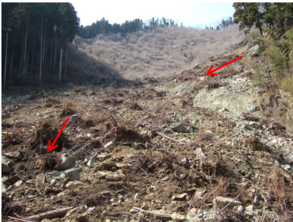
Photo 3.3.1.25 The left side valley and the joint
