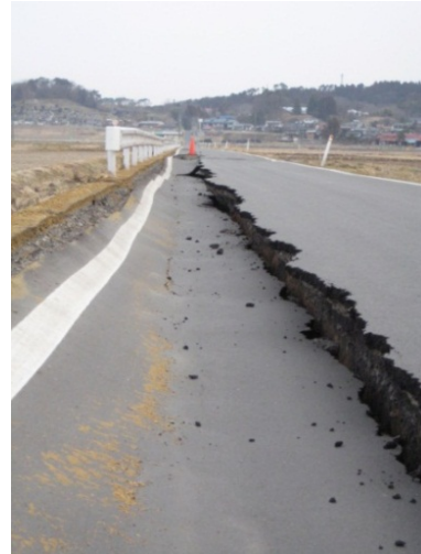
Photo 3.3.2.3 Conventional construction (without any anti-liquefaction measure)
