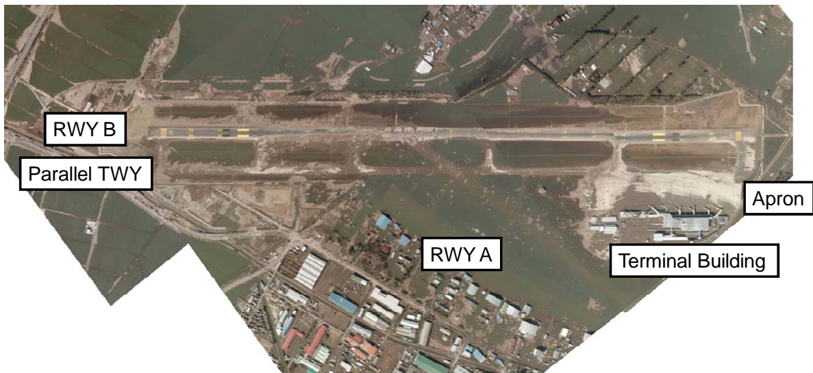
Photo 3.3.8.1 Situation at Sendai Airport around 14:00 on March 12, 2011 (photograph by the Geospatial Information Authority of Japan)
