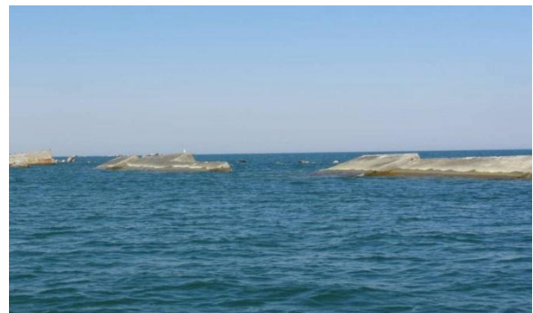
Photo 3.3.7.1 Soma port breakwater devastation state
