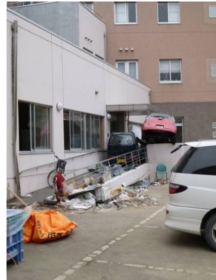
Photo 3.3.1.19 The south side wall of the elderly welfare center
