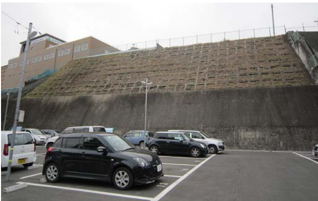
Photo 3.3.1.7 Retaining wall, cribwork (no anomaly seen on retaining wall)
