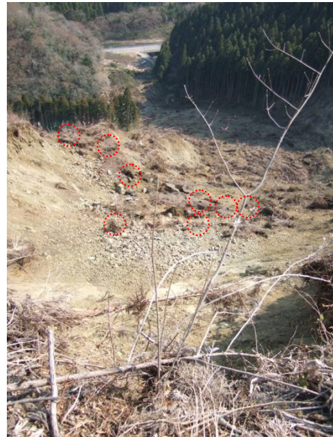
Photo 3.3.1.30 Stubs left close to the top (seen from the top)
