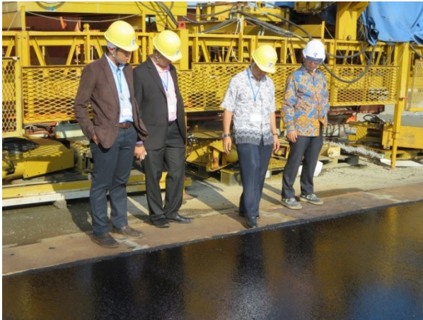
Trial construction of AsButon Guss asphalt
