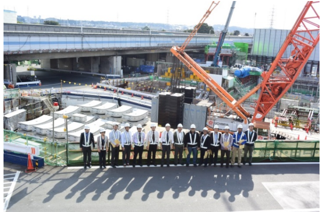
Construction site of Tokyo outer Ring Road
