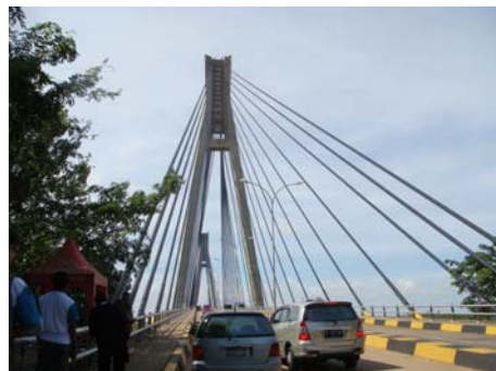
(Balerang Bridge Site Observation)
