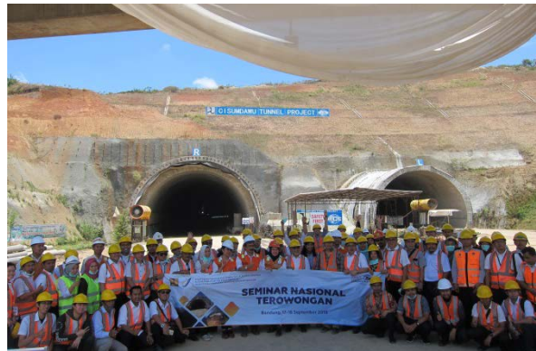
Site visit on the road tunnel construction
