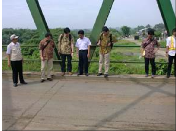
Discussion in the trial construction site
