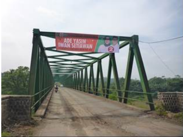
Cisadane Bridge (The trial construction site)
