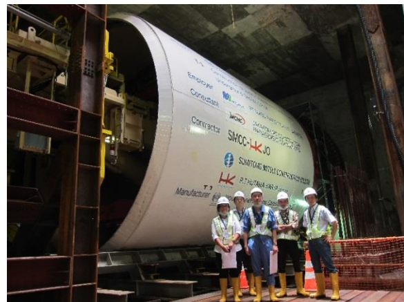
Site Visit to Construction Site of Japanese private company
