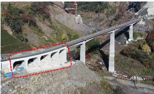
Aso Chōyō Ōhashi after completion of recovery
