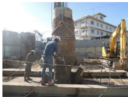
Photo. How the piles were removed on our investigation site
