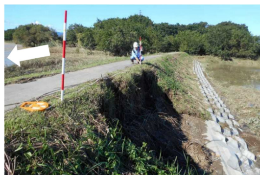
Photo 1: An example of back slope erosion at a site where crisis management-type structural countermeasures were used (left bank of 6.2 kp of the Toki River in the Arakawa River system)
