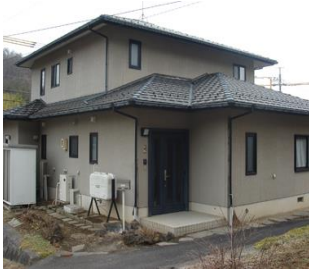
Photo 2-1: A properly managed vacant house
