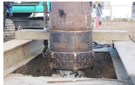
Photo 1: Removal of existing piles in the experiment
