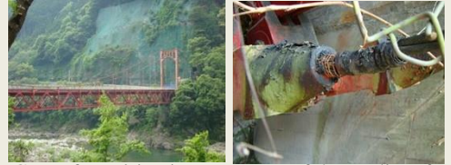
Case of requiring improvement of the quality of periodic inspection (For suspension bridges, it is difficult to grasp the condition of cable under covering only with proximity distance observation)
