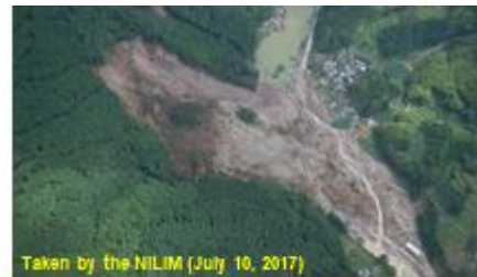
Oblique photo of slope collapse (July 2017 Northern Kyushu Heavy Rain, Hita-shi, Oita)
