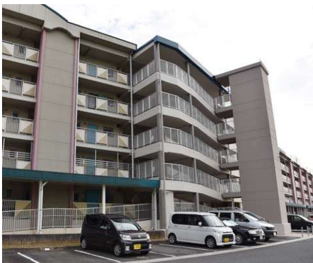
Photo 1: Installation of an elevator between two buildings (public rental housing)
