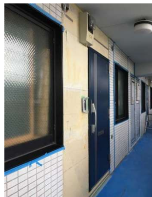
Photo 2: Improved insulation performance using exterior insulation + double sashes (private condominium)
