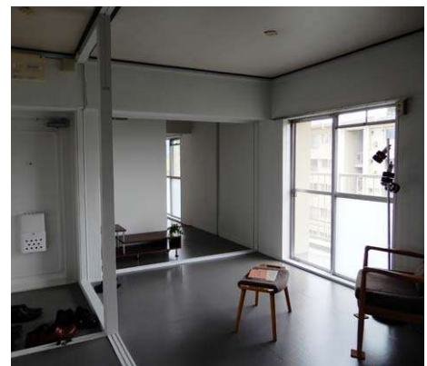
Photo 3: Expansion of living space by combining two units into one (public rental housing)
