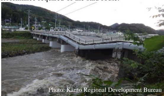
Photo: Hounji Bridge on National Highway No. 20 where subsidence of the bridge pier occurred
