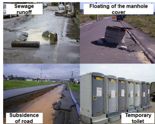
Photo: Example of sewerage facility at the time of disaster
