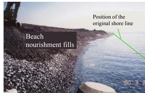
Photo: Gravel nourishment in Fuji Coast, Shizuoka
