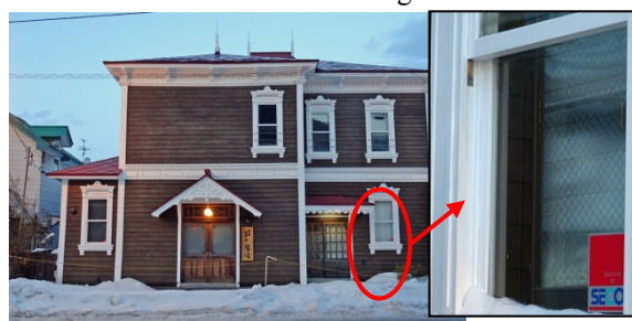
Photo 3. An example in which wire glass is used on the inside of an opening
