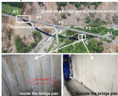
Photo: Conditions of major damage on Aso Choyoo Bridge
