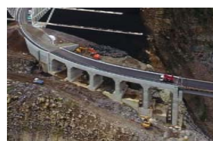
(a) Recovery with multiple RC reinforcement structure
