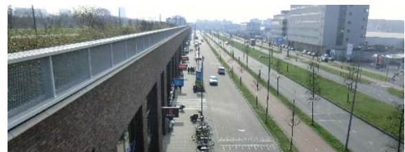
Photo 1: Development of a park (upper section) and stores (lower section) that function as a levee in Rotterdam, the Netherlands
