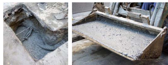
Figure 3. Backfilling using low-strength concrete (Taiwan)
