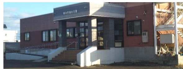
Photo 3: Raising of the foundation of buildings in high-risk areas in the city of Sapporo
