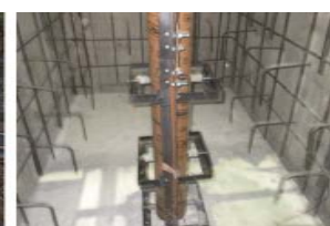
(b) Recovery with concrete filling
