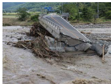
Photo 1: Road bridge of a national road damaged in a flood
