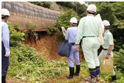
Photo 2: On-site inspection at Noboritani Snow Shelter
