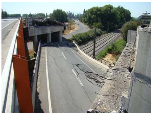
Photo 1 Bridge unseating during the 2010 Chile earthquake
