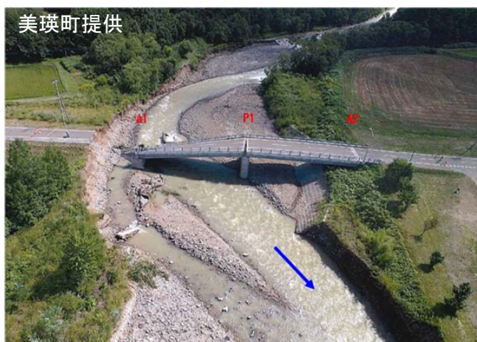
Fig. 1 Damage to Kyusen Bridge (Bebetsu River, Hokkaido)
