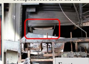
Conveyors blocking the closing motion
