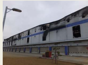
External appearance of the building after the fire
