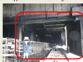
Malfunction of fire shutters
