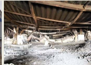
Collapsed roof due to the fire
