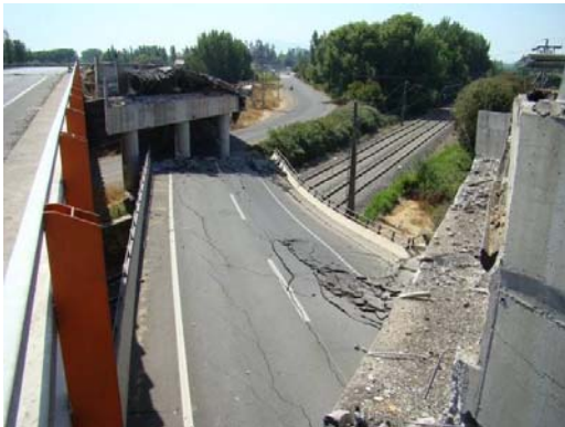
Photo 1 Bridge unseating during the 2010 Chile earthquake
