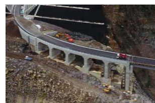
(a) Recovery with multiple RC reinforcement structure
