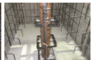
(b) Recovery with concrete filling
