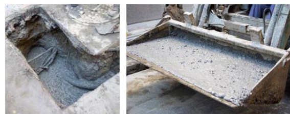
Figure 3. Backfilling using low-strength concrete (Taiwan)
