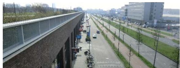
Photo 1: Development of a park (upper section) and stores (lower section) that function as a levee in Rotterdam, the Netherlands
