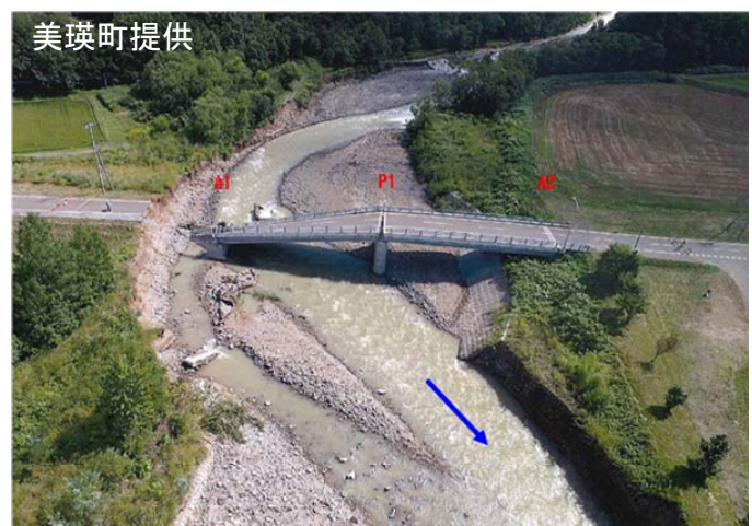
Fig. 1 Damage to Kyusen Bridge (Bebetsu River, Hokkaido)
