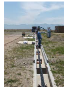
Test of laying cables in a compact box
