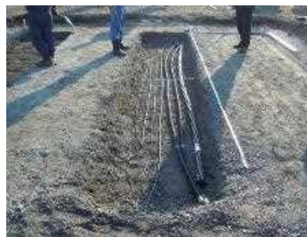
Checking damage to underground cables
