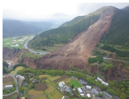
Large-scale slope failure triggered by the earthquake (2016 Kumamoto Earthquake)
