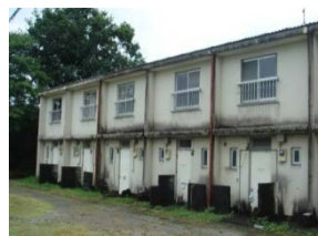
Photo 3: A deteriorated building in an existing public apartment complex to be demolished.
