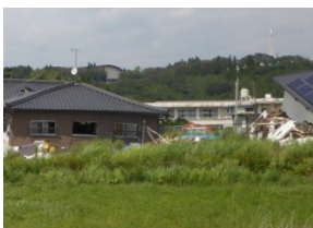
Photo 1: Damaged houses in a community
