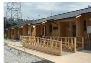
Photo 4: Wooden temporary houses that have the needs as permanent houses.
