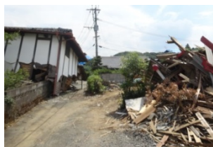
Photo 2: Damaged houses in a community
