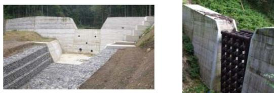
Figure 2 Sabo dam (Left: Impermeable type, Right: Permeable type)
