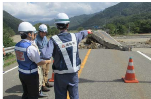
Photo 1: On-site study being conducted at Chiroro Bridge (National Route 274)
