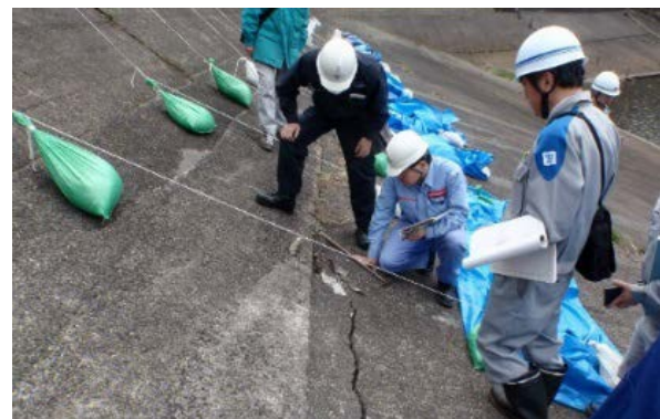
Photo 2: Investigation of Jizobaru Dam (Upstream face of the dam body)
