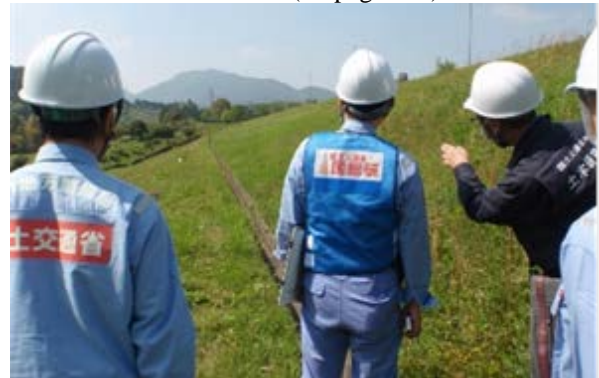
Photo 1: Investigation of Midorikawa Dam (Downstream face of the side dam)
