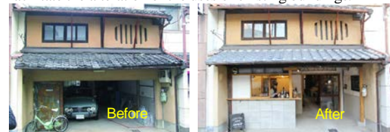
Photo 3: Example of Alteration of Building Use from House to Restaurant/Store
