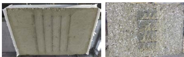
a) Immediately after fire b) Several days after fire Figure 2 Conditions of concrete after fire
