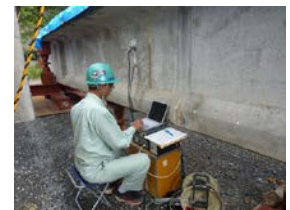
Photo 3: Example of a test to check applicability to an actual structure
