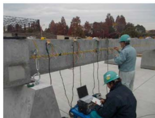
Photo 1: Nondestructive investigation underway
