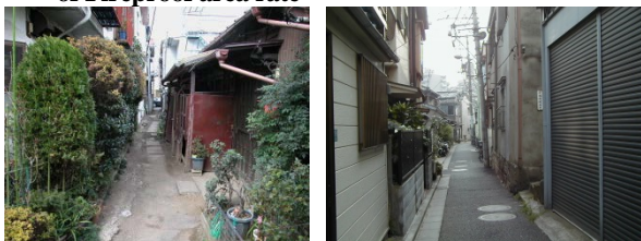
Photo 1. Conditions of densely built-up areas with high fire risks
