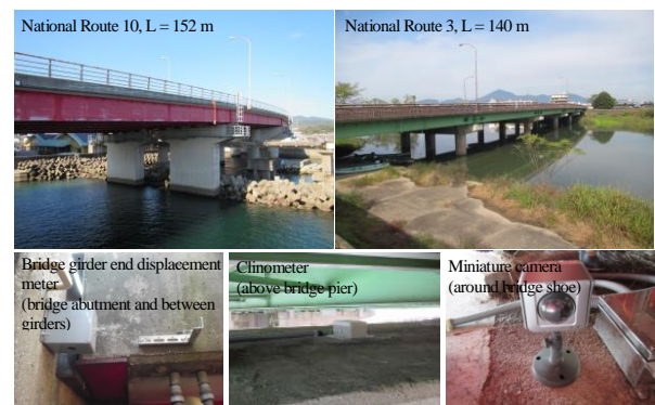
Figure 2 Bridges that were newly installed (Upper photos) and sensor installation examples (lower photos)
