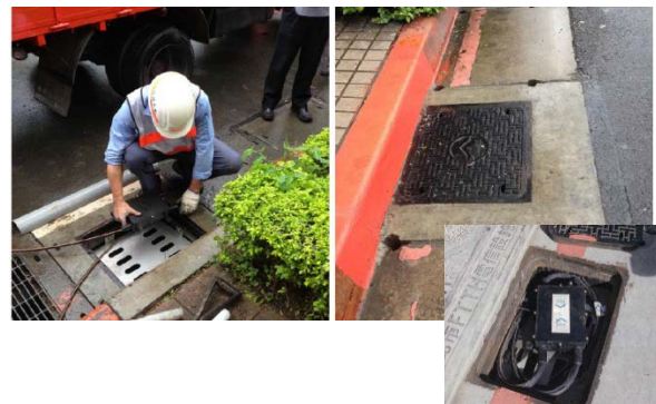
Figure 1: Laying of communication lines utilizing street gutter (Taiwan)
