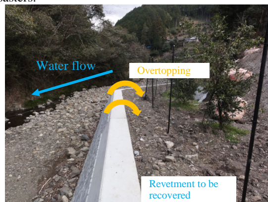
Photo 1: Recovery from the damage in the inner side of the bend
