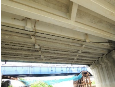
Photo 1: Reinforcement of bridge with external cables
